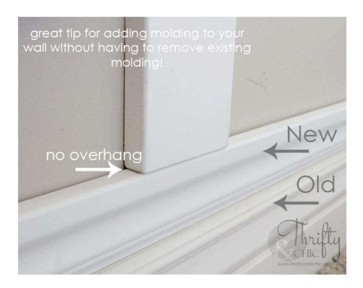
Here's the same concept, but with a smaller transition piece. You can install this transition piece right on top of the baseboard, as well.
