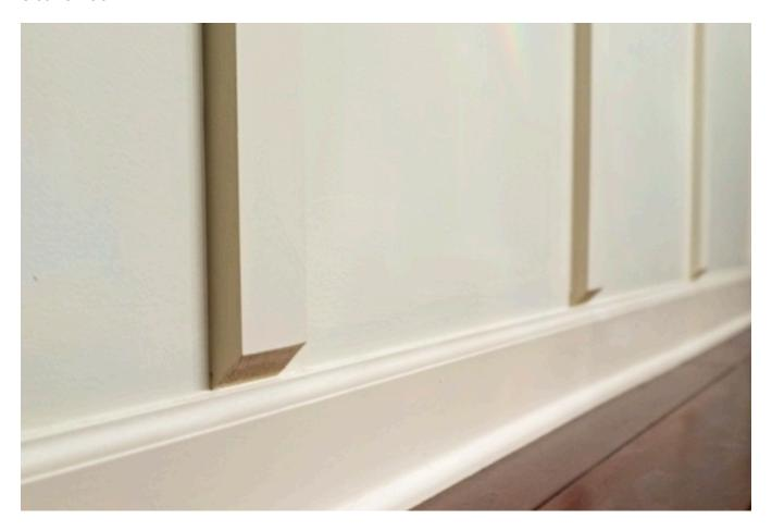
Here's a pic of both options side by side. In this case, they chose to go with the thinner wood rather than cut at an angle.
